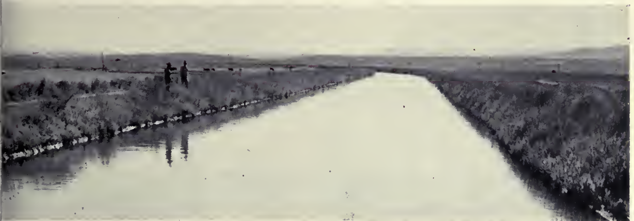
EXCELLENT GRASS COVER on canal and lateral banks of the North Unit, Deschutes project, in Oregon prevents weed infestations.
